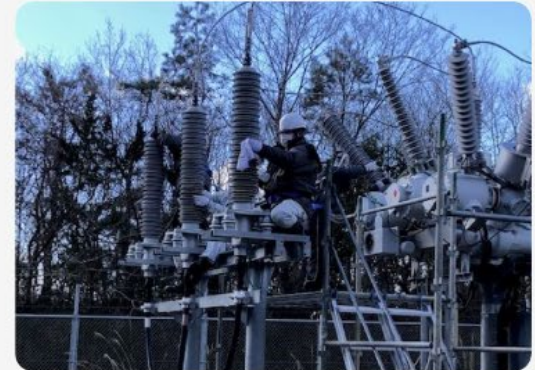
CH Hindrance inspection
