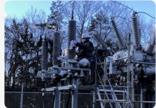
CH Hindrance inspection
